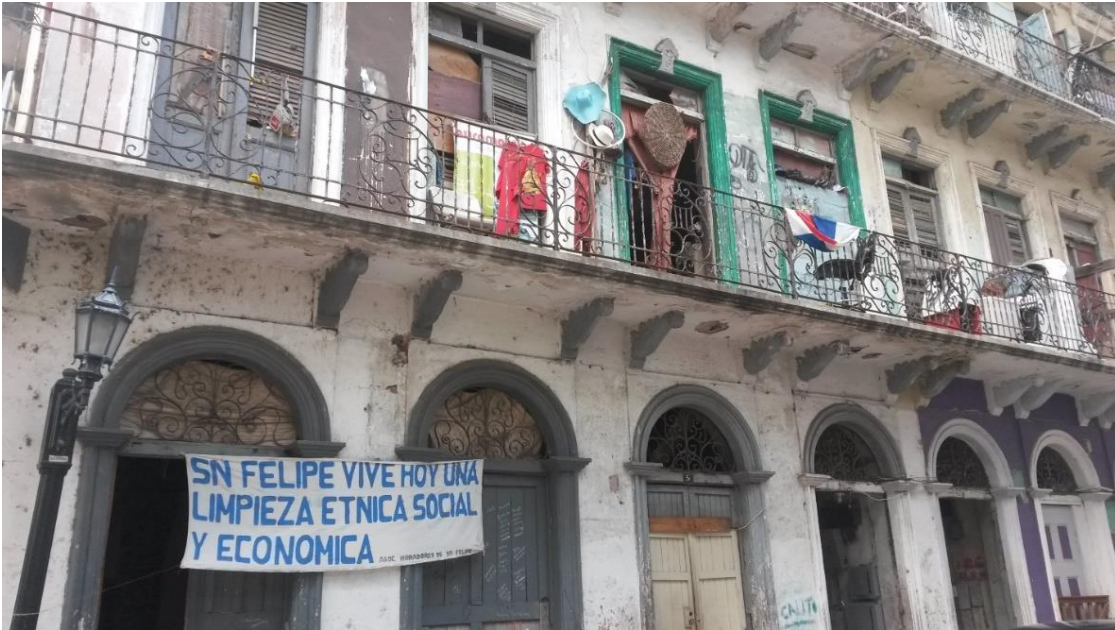
Figure 2.10: Occupied unrestored building in San Felipe
