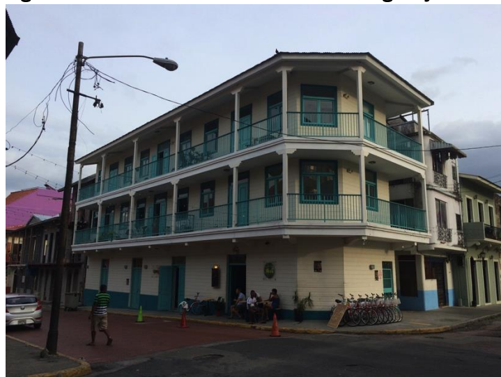
Figure 6.2: Conservatorio Affordable Housing Project
